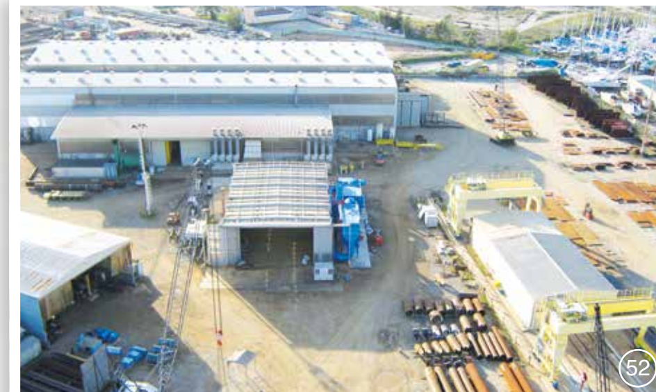
Filtro autopulente e impianto recupero sabbie Automatic sleeve filter unit and recovery sand plant
