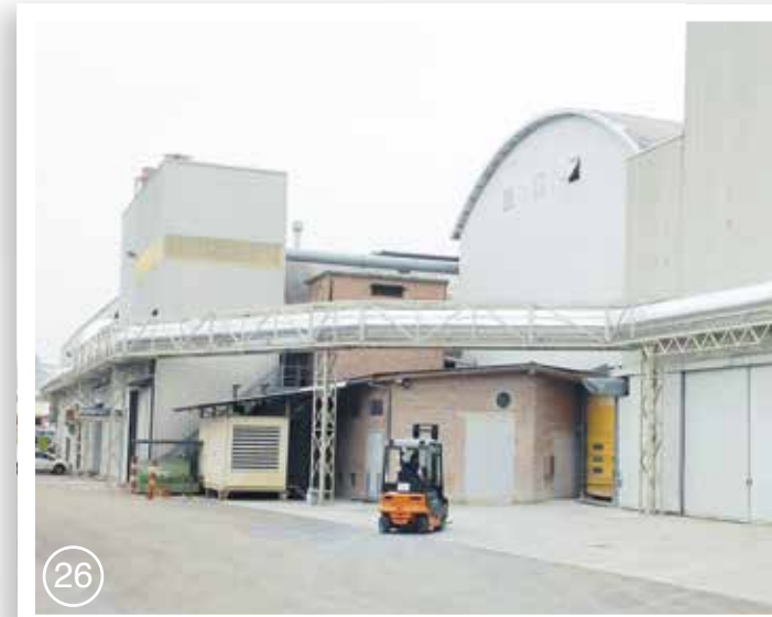
Collettore coibentato per recupero termico ATM Insulated pipeline for spray dryer's heat recovery system
